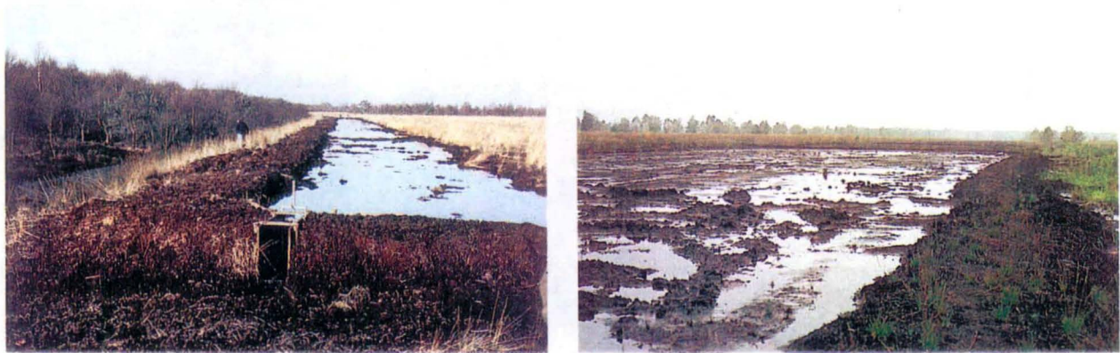
Shallow peat bunds forming lagoons within former peat workings at ( left ) Esterwege Dose (Germany) and ( right ) Kendlmühlfilze (Germany).
