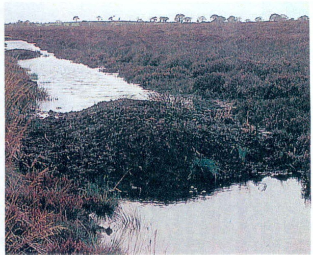
(b) Peat dams across wide drainage ditch; Wedholme Flow (Cumbria).
