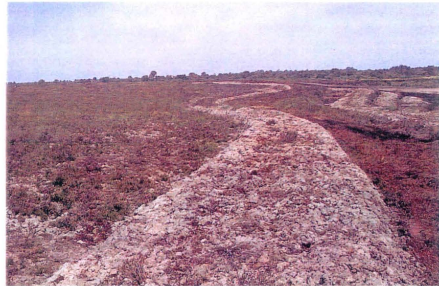
Plate 8.3 Scheme to protect an ancient wooden trackway within a raised-bog remnant at Corlea (Co. Longford, Ireland) (see Wynne & O'Donnell, 1993). Diagrammatic sketches of project layout and embankment (bund) construction and photograph of the bund (the remnant peat block is on the left of the photograph). [Sketches reproduced by permission of Bord na Mona]
