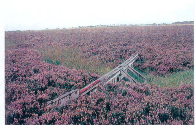
(f) Palisade timber dam across broad erosion gully; Blawhorn Moss (Lothian).
