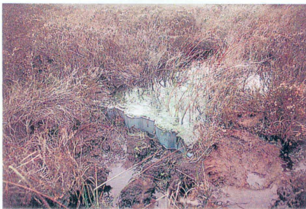
(c) Sheet-metal dam across narrow drainage ditch, Glasson Moss (Cumbria).
