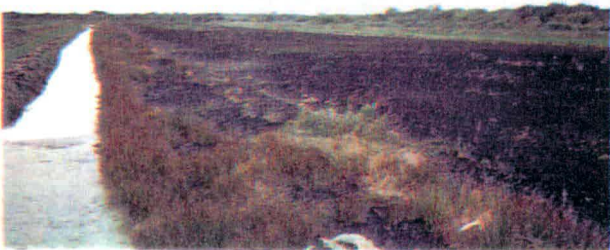
Plate 5.1 Getty's Mire, Somerset Levels. Former peat workings mechanically contoured to the predicted shape of the 'groundwater' mound [see text].
