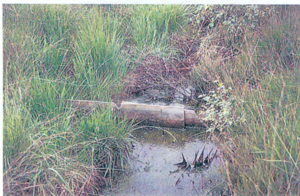
(e) Simple plywood-sheet dam across narrow ditch; Danes Moss (Cheshire).
